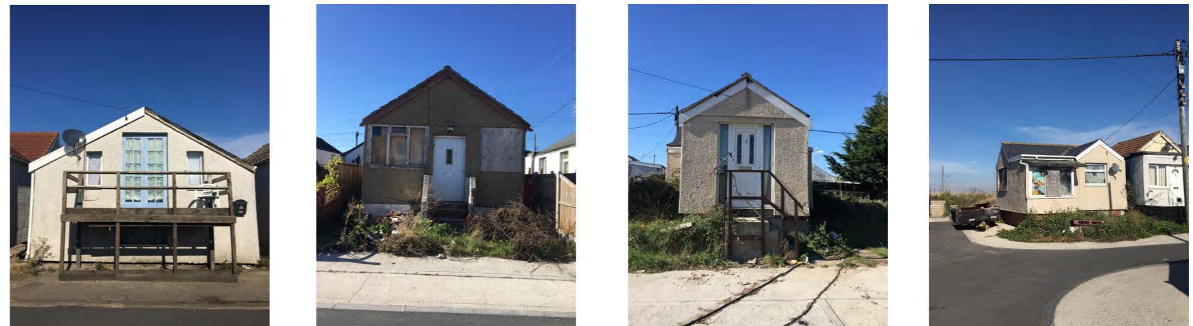
Fig. 39. Examples of occupied housing in very poor condition.
